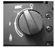
To turn to the PILOT position from the HIGH or LOW positions, press the control knob in, and return to the pilot position and release.
